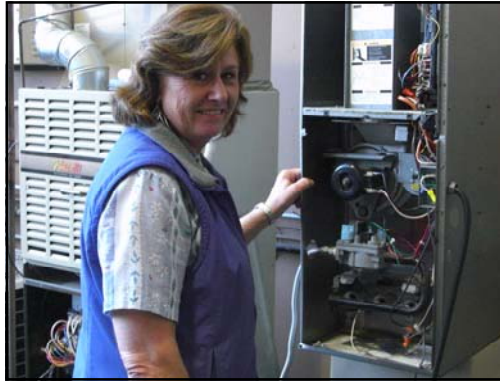
Gail Mathis working on a home heating unit.
